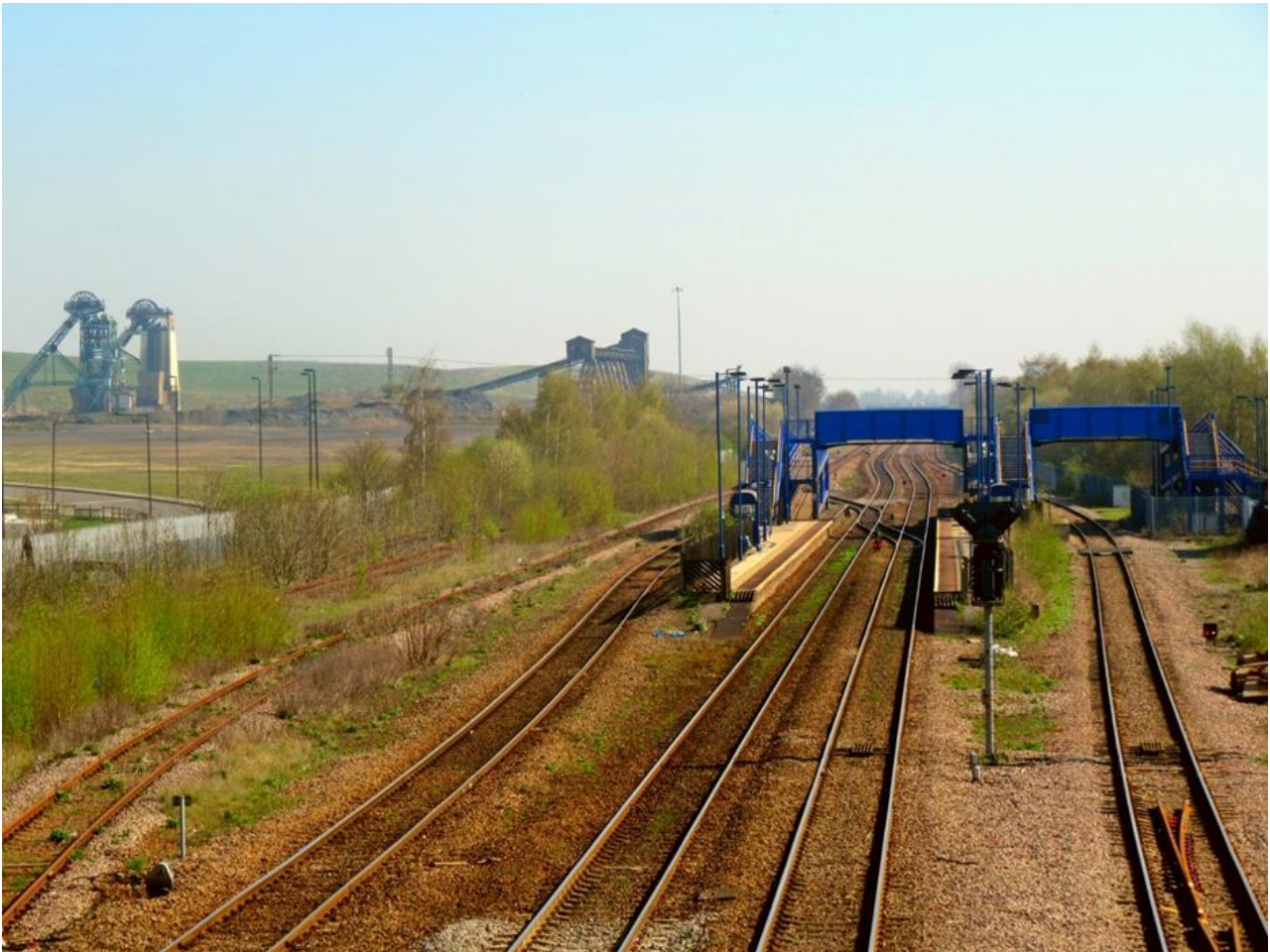
Hatfield and Stainforth Railway Station (Right) with Hatfield Main Colliery Head Gears and Conveyor system (Left), Stainforth
